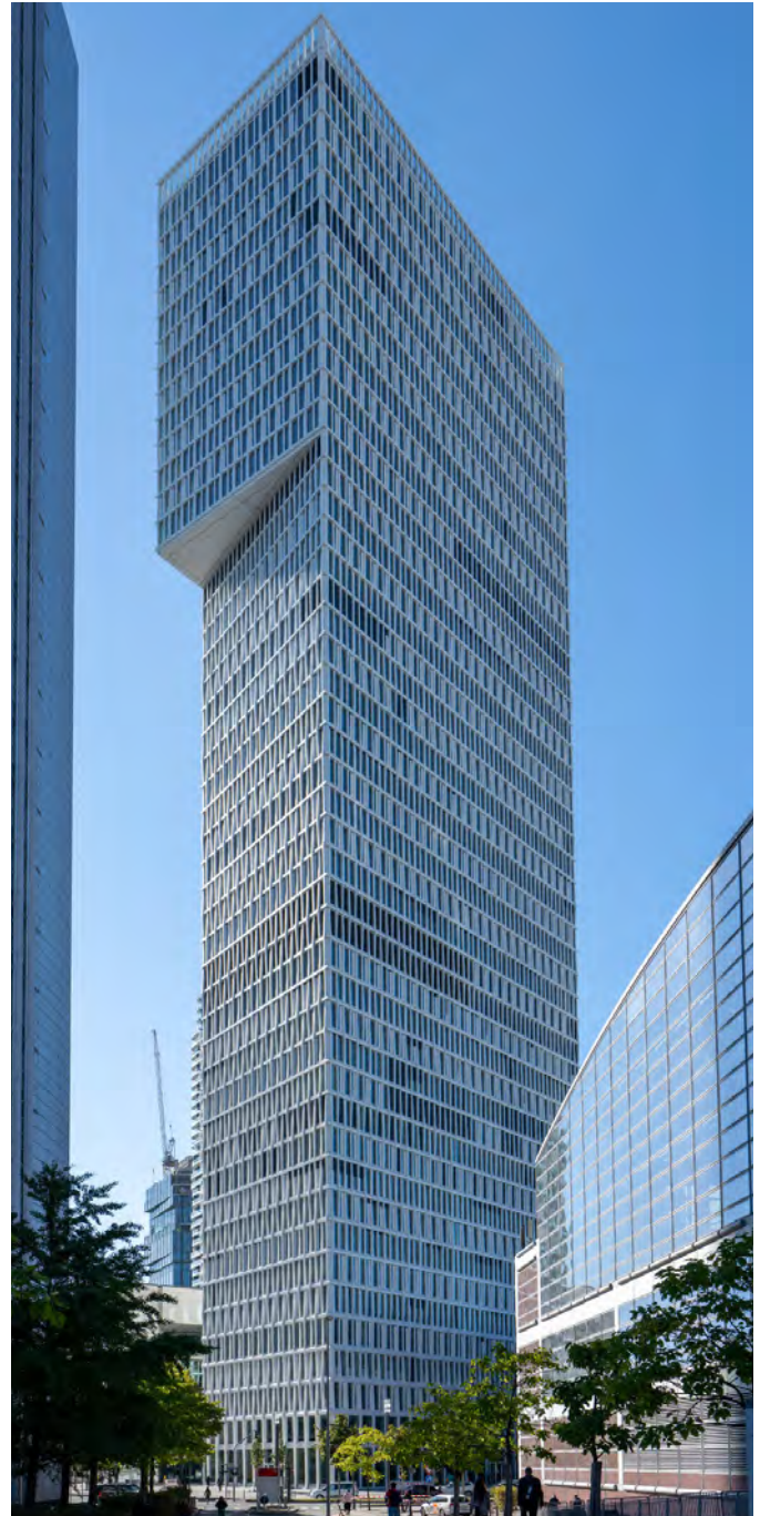
The finished construction of ONE at Frankfurt am Main, Germany
