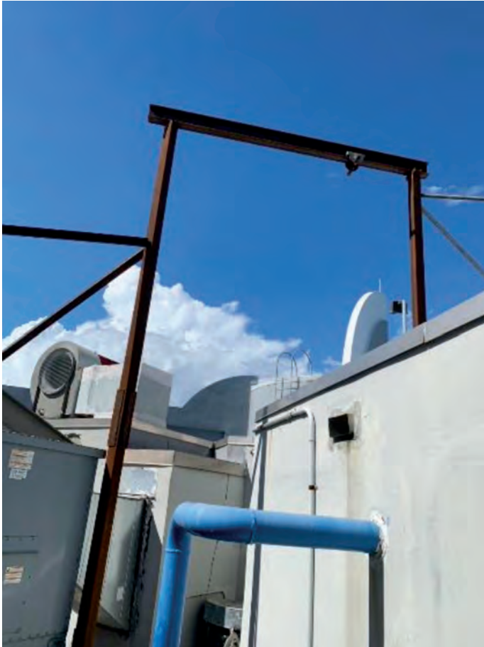
Special rigging was vital to the project's success.
