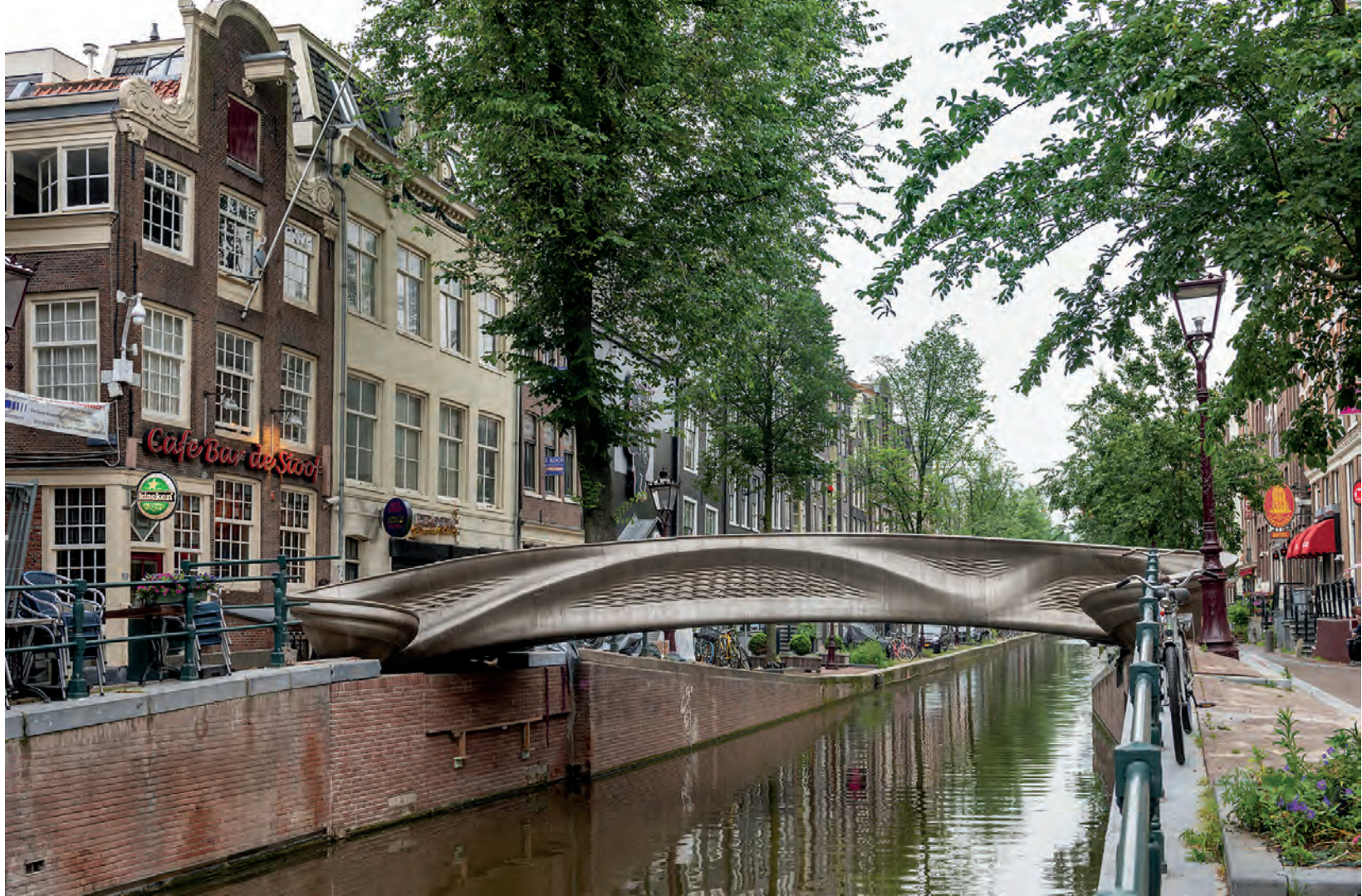
Steel bridge in the city center of Amsterdam, The Netherlands, “printed” by MX3D; courtesy of MX3D
