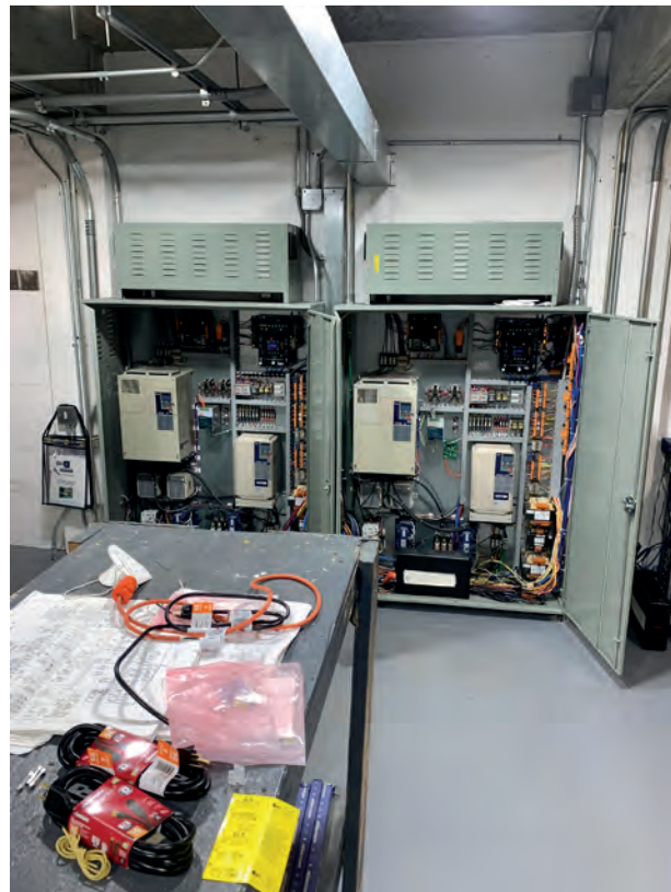
Suncoast replaced all components in the machine room.
