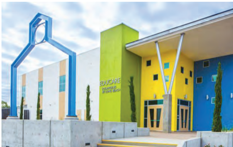
A bright green modular elevator at Educare Los Angeles at Long Beach; photo courtesy of MEM
