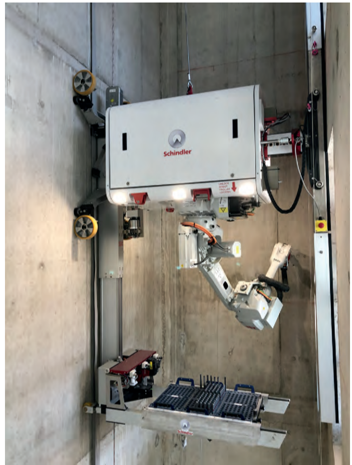
Installation robot Schindler R.I.S.E at work; courtesy of Schindler
