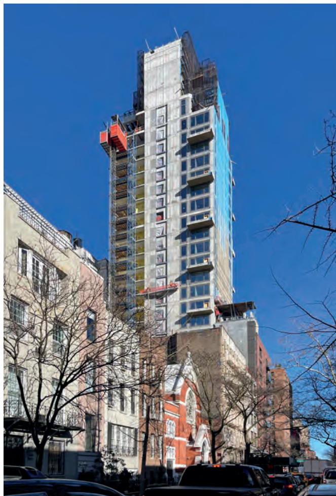
In March, the final set of balconies along the northern corner of the tower on 249 East 62nd Street was yet to be built, and will probably have to wait for the construction elevator to be disassembled; photo by Michael Young for New York YIMBY.
