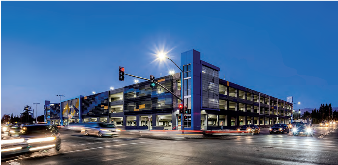
Multi-level parking structure at San Jose State University's south campus; photo courtesy of Jason O'Rear for Watry Design, Inc.
