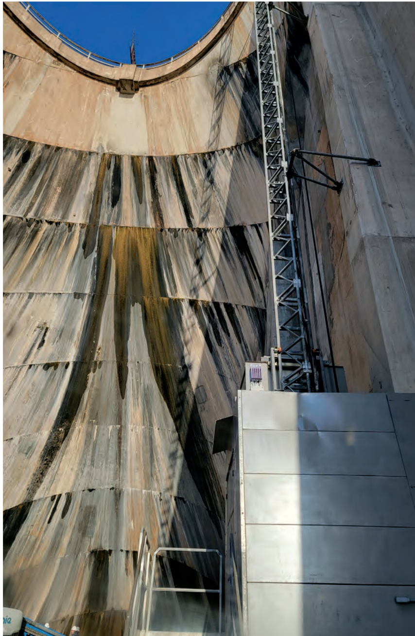
Rack-and-pinion elevator on a hydroelectric dam
