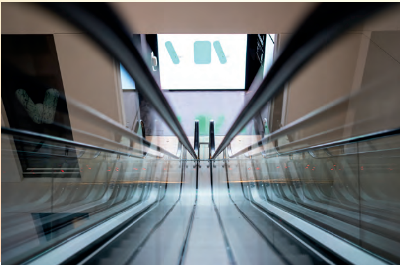
The escalator step width is 600 mm, and the height of the balustrade is 1100 mm.
