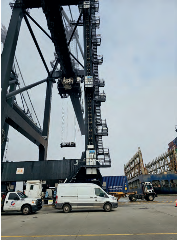
Container crane personnel elevator
