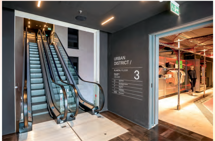
A total of 15 escalators and elevators were installed by TKE.
