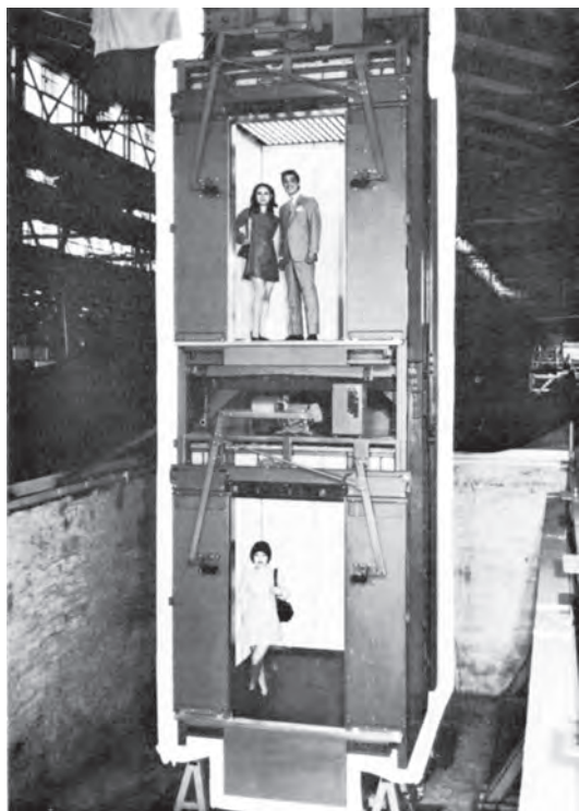
Figure 3: Mitsubishi Electric Company Ltd. double-deck elevators as seen in their factory
